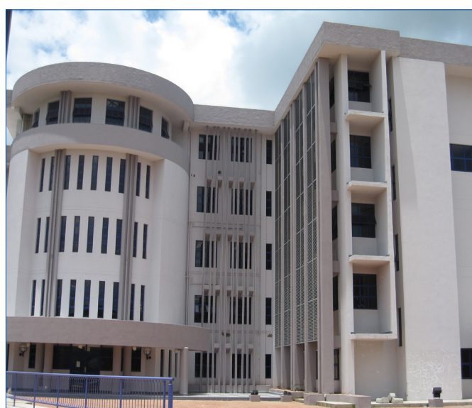
Figure 4.1: New laboratory complex, Mbabane, Swaziland
