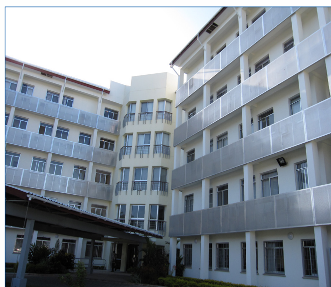
Figure 4.2: New laboratory complex, Dar es Salaam, Tanzania
